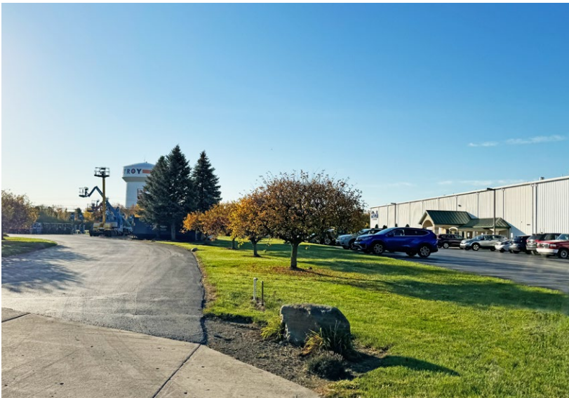
FIGURE 37: EXAMPLE OF LIGHT INDUSTRY STRUCTURES
