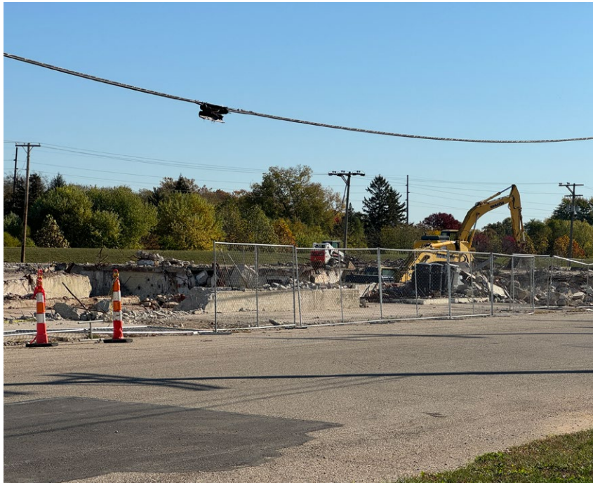
FIGURE 78: DEMOLITION OF THE FORMER SPINNACKER BUILDING
