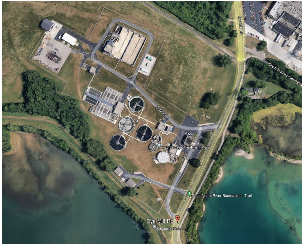
FIGURE 65: TROY'S SANITARY SEWER TREATMENT PLANT
