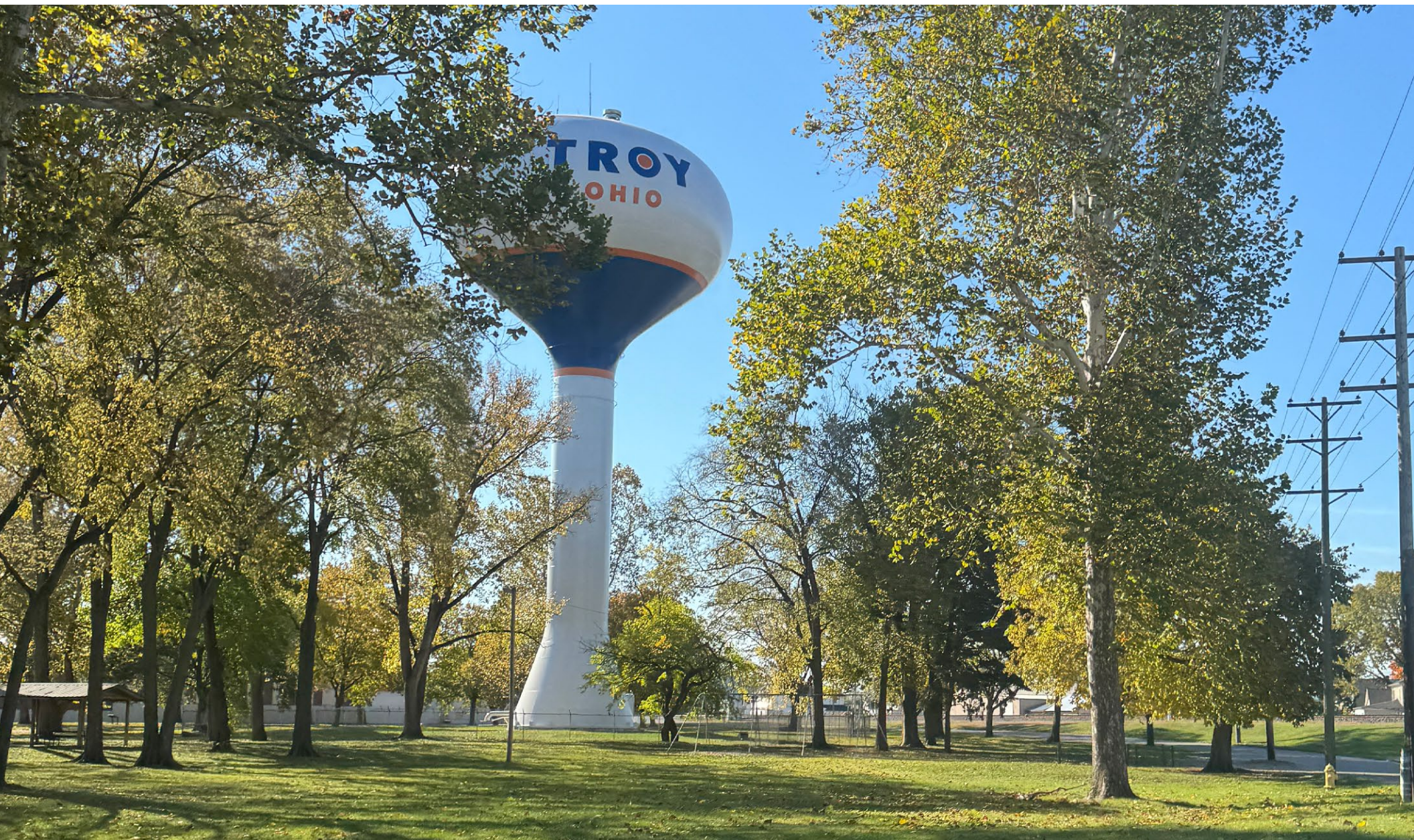
FIGURE 40: AN ELEVATED WATER TANK IS AN EXAMPLE OF A UTILITY LAND USE
