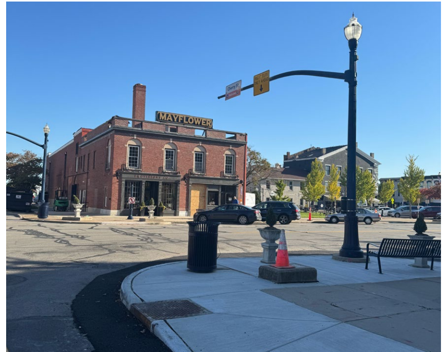
FIGURE 79: RENOVATION OF THE FORMER MAYFLOWER BUILDING
